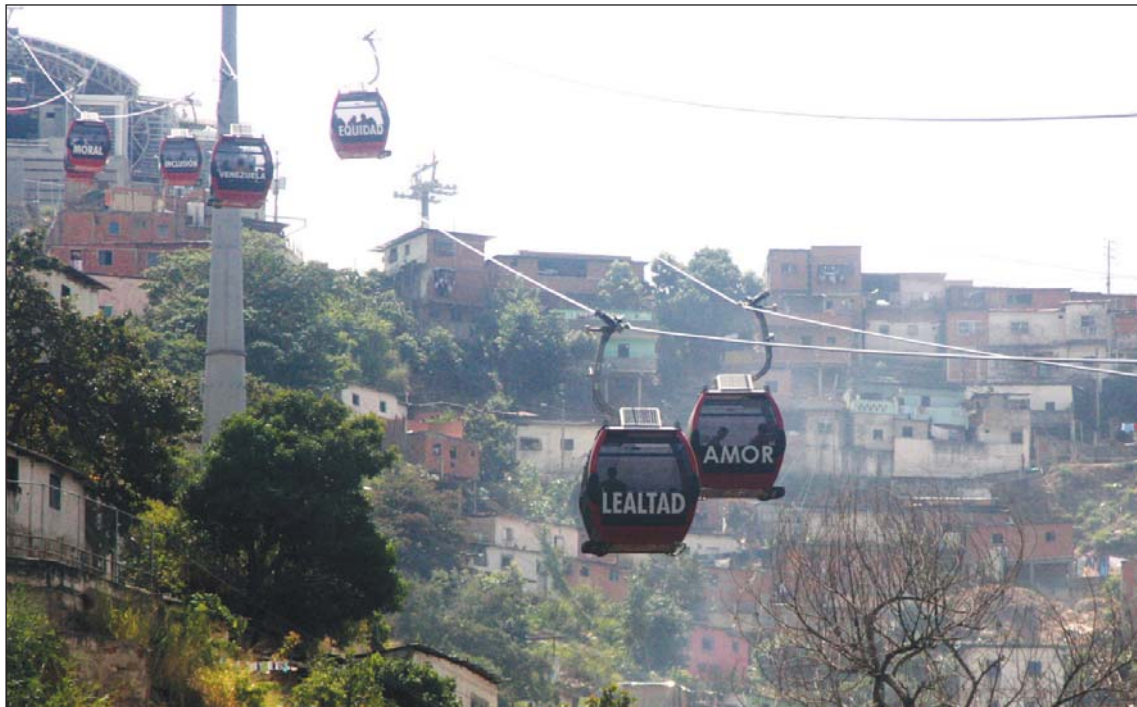
The new Metrocable system will bring relief to a poor community with homes in areas difficult to reach by vehicle
